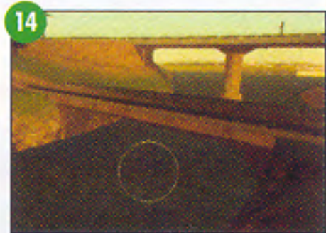
14 Under the bridge, North West of Palomino Creek.
