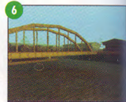
6 Under the docks bridge, situated on the small "island" part of the Docks.
