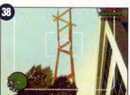
38 The structure at the top of Missionary Hill.
