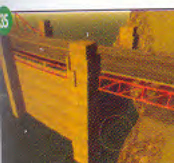
Between the Gant Bridges northern most support and a cliff.
