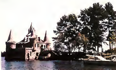
The power generator of Heart Island Castle is a miniature version of the main castle located nearby.
