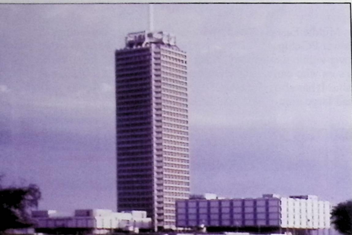
The World Trade Center building in Dubai
