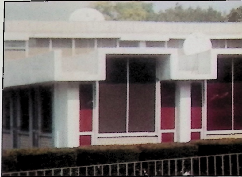
Satellite dish atop Clinton High School
